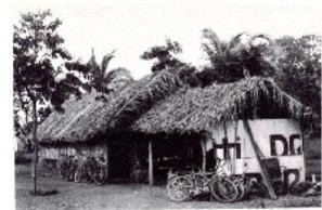
Figure 1 Houses made of barroite covered with babassu straw. Source: Caixa Econômica Federal
